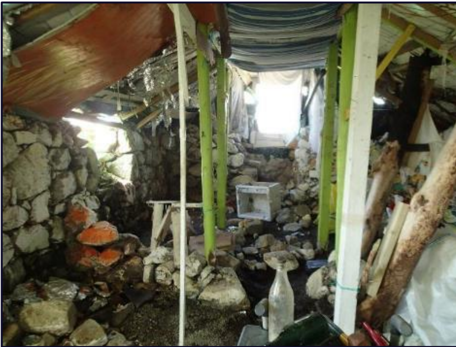
Figure 21: West Gable, interior
