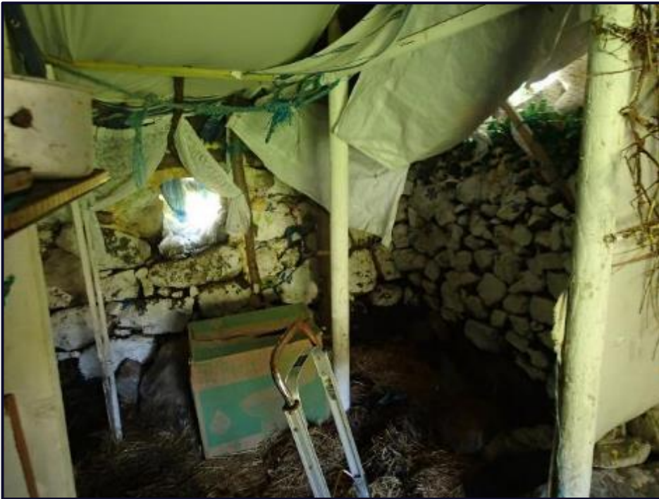
Figure 19: South wall, east end, interior
