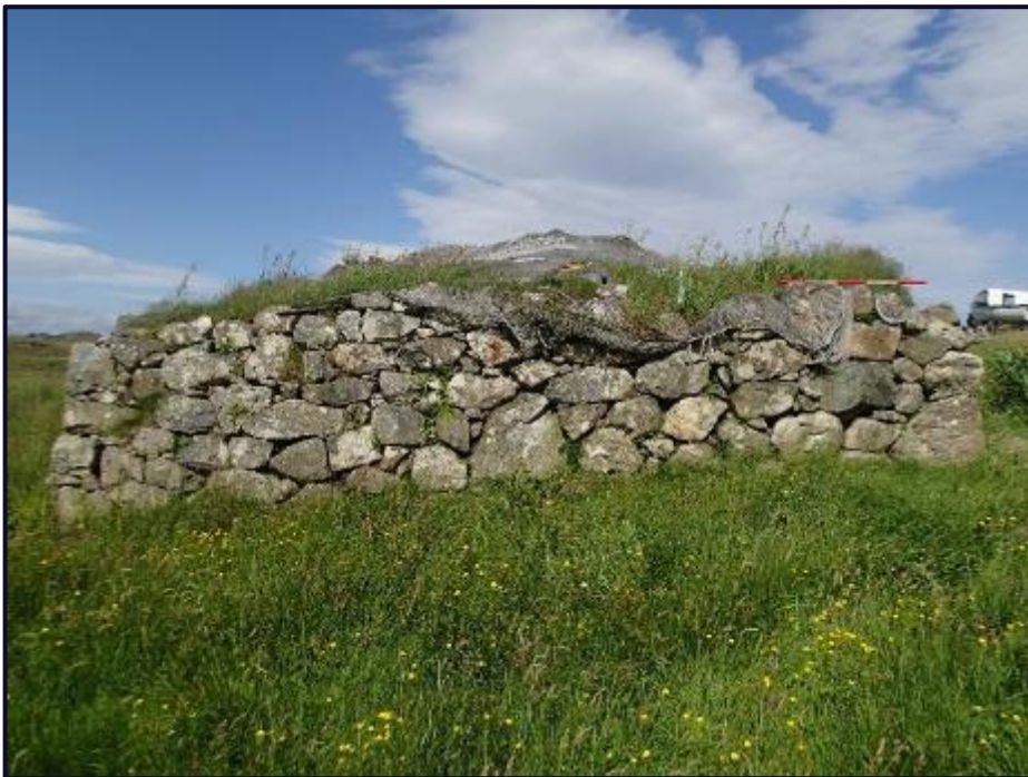
Figure 11: East Gable. The large stone in the centre is a lintel for the drain.
