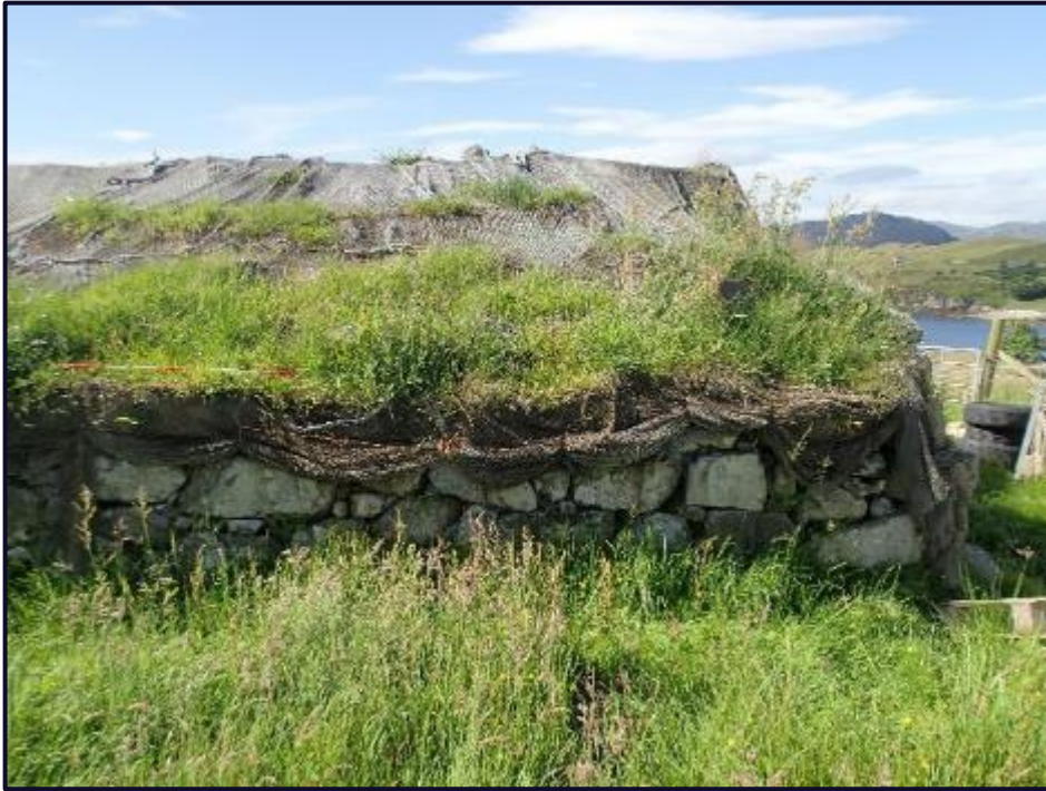
Figure 16: North side, west end
