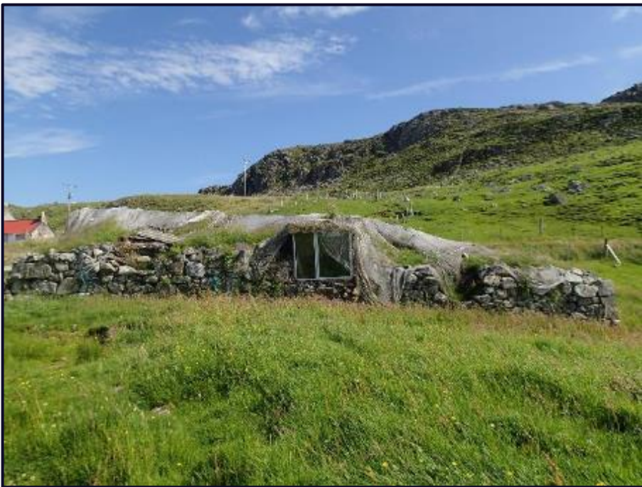
Figure 13: South wall with windows
