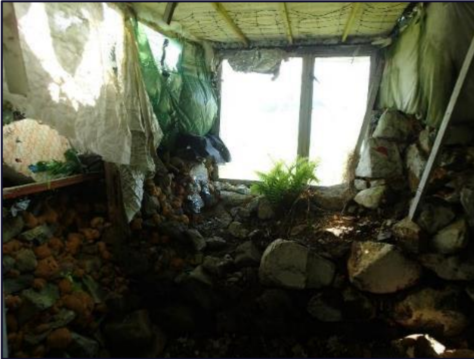
Figure 20: Central window in South wall, interior
