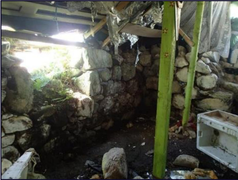
Figure 22: Western window, south wall, interior
