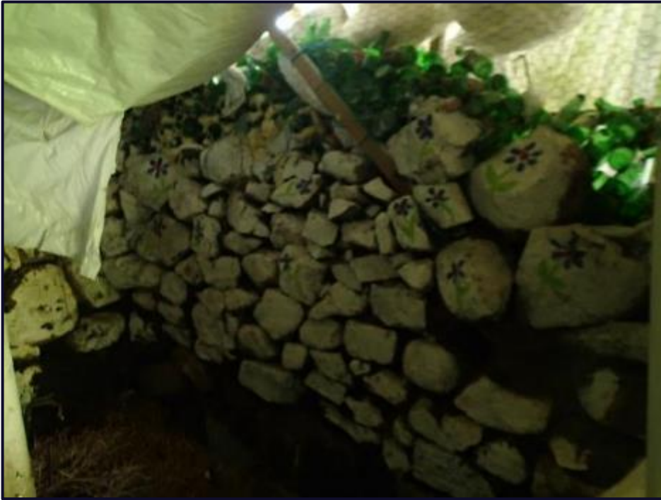
Figure 18: East gable, interior
