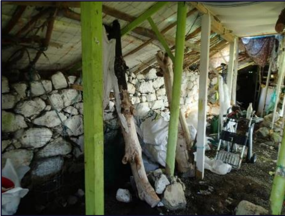
Figure 24: North wall, interior
