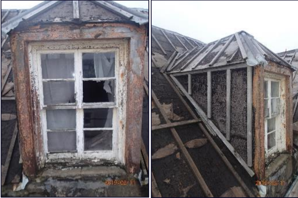
Figure 13: Dormers on Keith St facade
