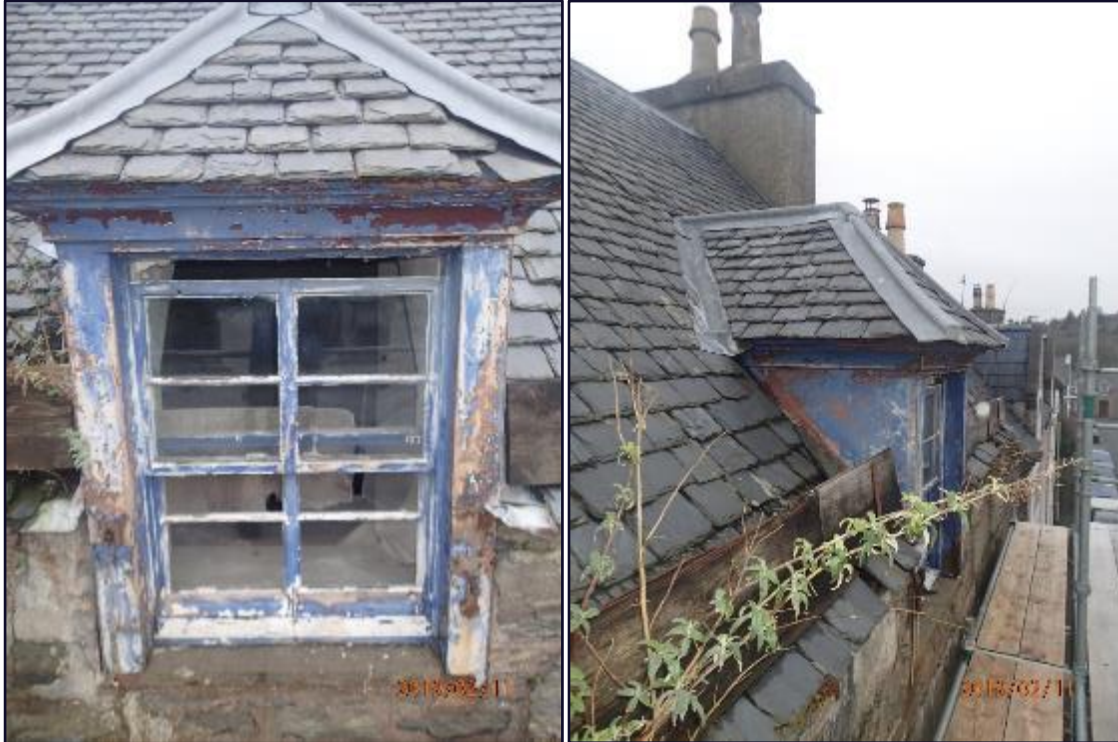
Figure 12: Dormers on Scotland St facade
