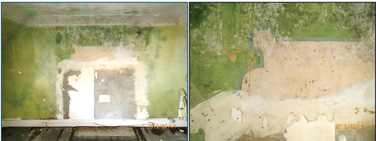
Figure 29: FF10 and decorative distemper painting around now blocked up hearth
