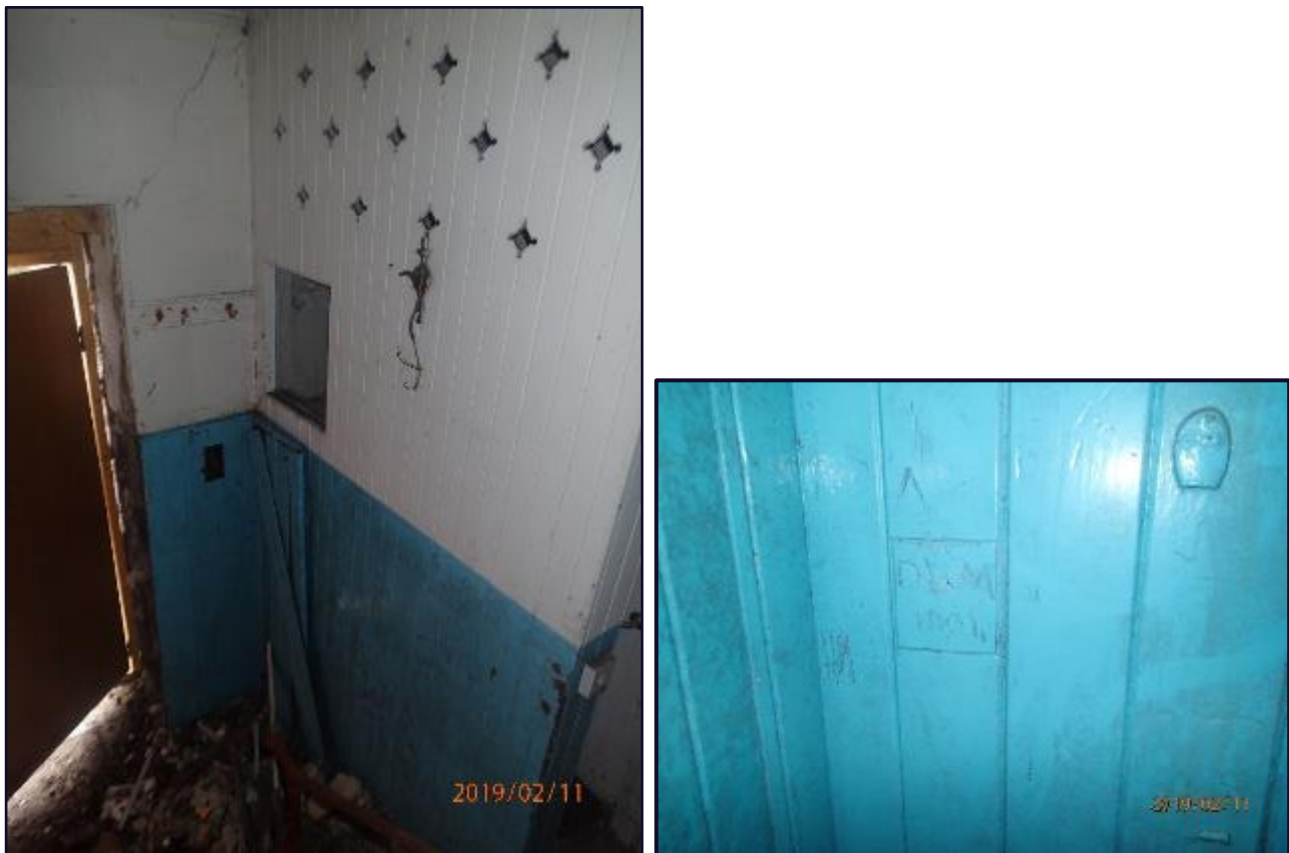
Figure 23: GF1 and GF2, showing decorative ventilation and graffiti
