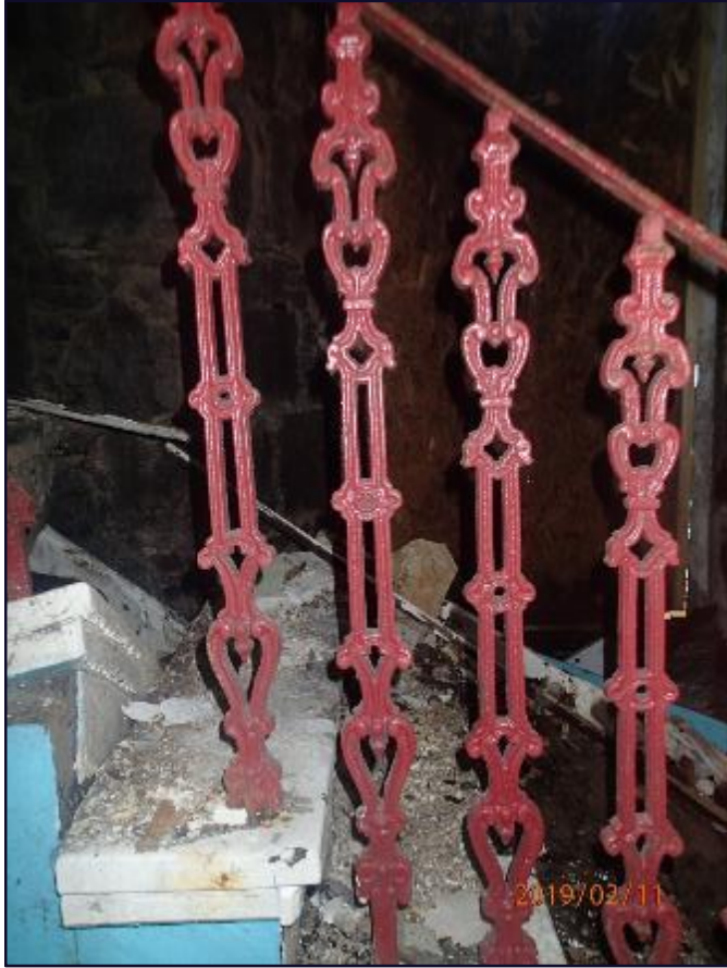
Figure 24: Decorative cast iron Banister supports
