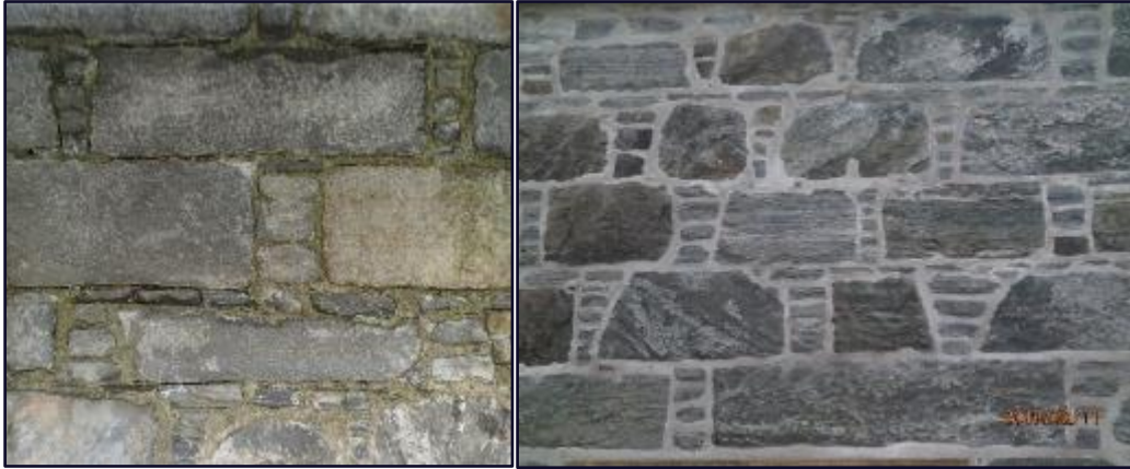
Figure 16: Decorative pinning stones, School wall to the left, Castle wall to the right
