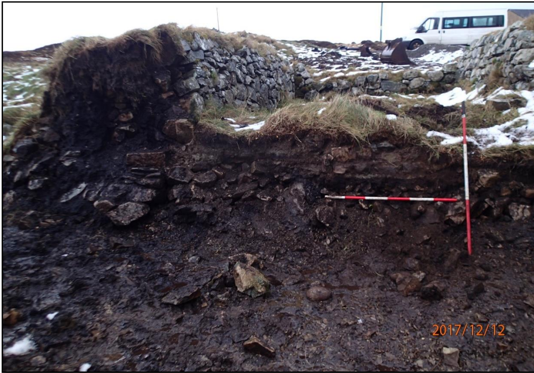
Figure 22: West side of main Blackhouse showing Peat core (003) in wall, internal stone facing (004) and occupation layers (009)/(011)
