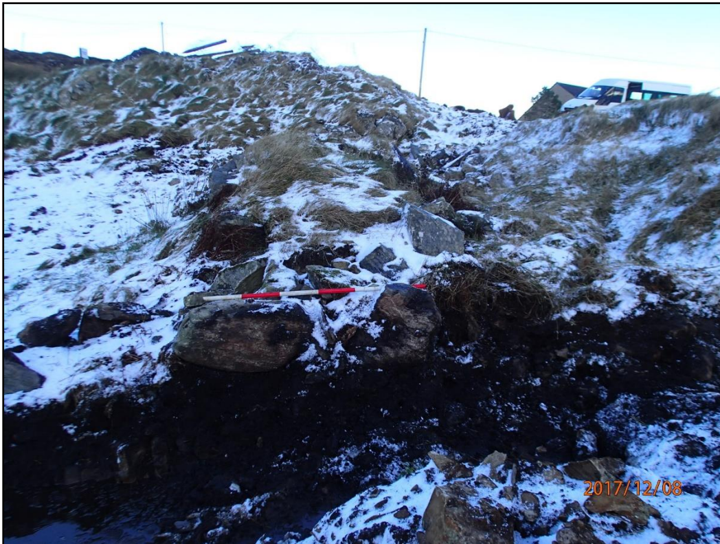
Figure 25: Barn wall sitting on (014) and Bedrock
