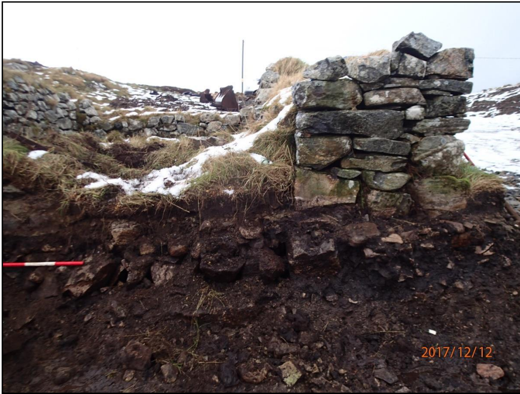
Figure 24: East wall (002)/(003) and foundations (007)/(008).
