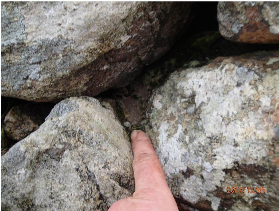
Figure 16: Clay pointing of internal walls
