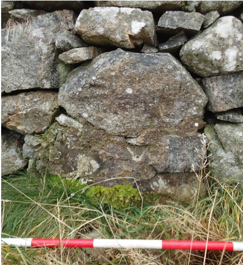
Figure 15: Concrete pointing of section of internal wall
