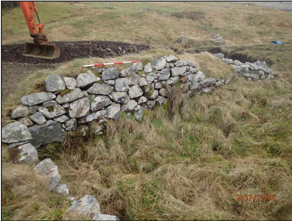
Figure 13: Northeast internal wall showing coursing
