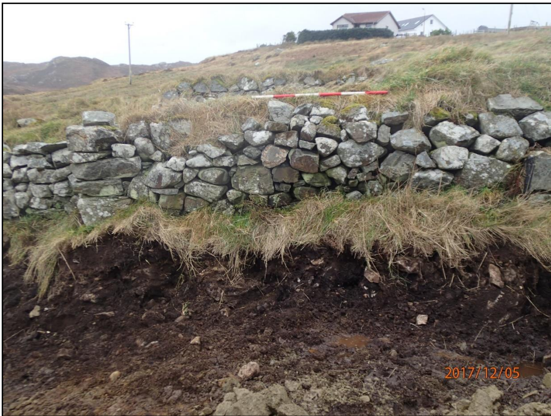
Figure 12: Northeast external wall showing random coursing
