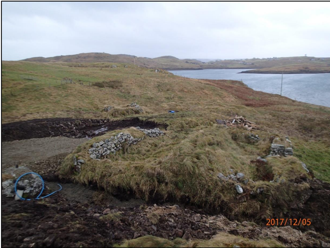
Figure 9: Looking South at Blackhouse and Barn. New access road to the left hand side.
