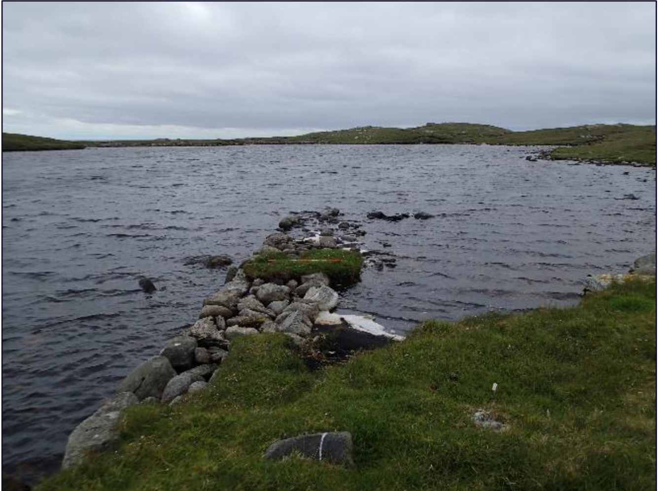
Figure 36: Water intake on Loch a Rudha Chaoil
