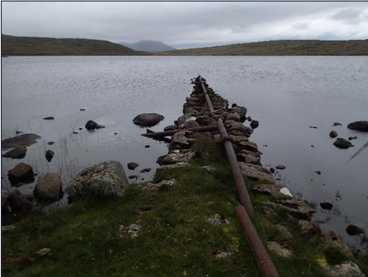
Figure 37: MOD water intake rig at Loch Mheacleit, c 1km to the south, for comparison with Site 6, above.
