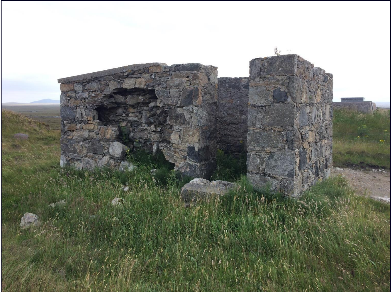
Figure 30: Second “look out” structure, Bru, West side, Lewis, facing south
