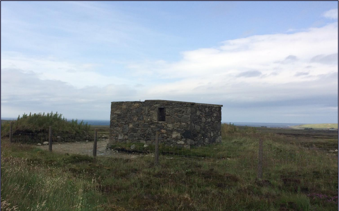
Figure 31: Second “look out” structure, Bru, facing north
